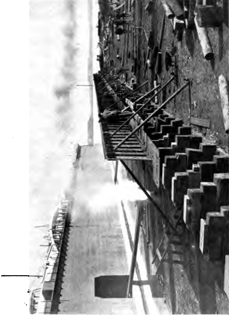
The First Step in the Making of a Ship—Laying the “Keel Blocks.”
